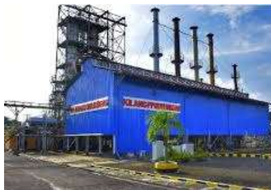
Gambar 1. Kilang PPSDM Migas
